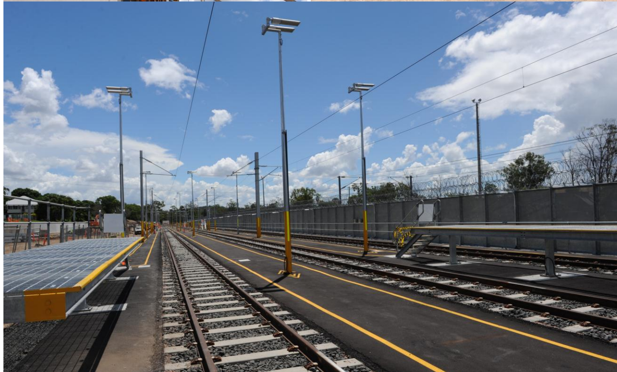
Top: Platform and services retaining wall and road
