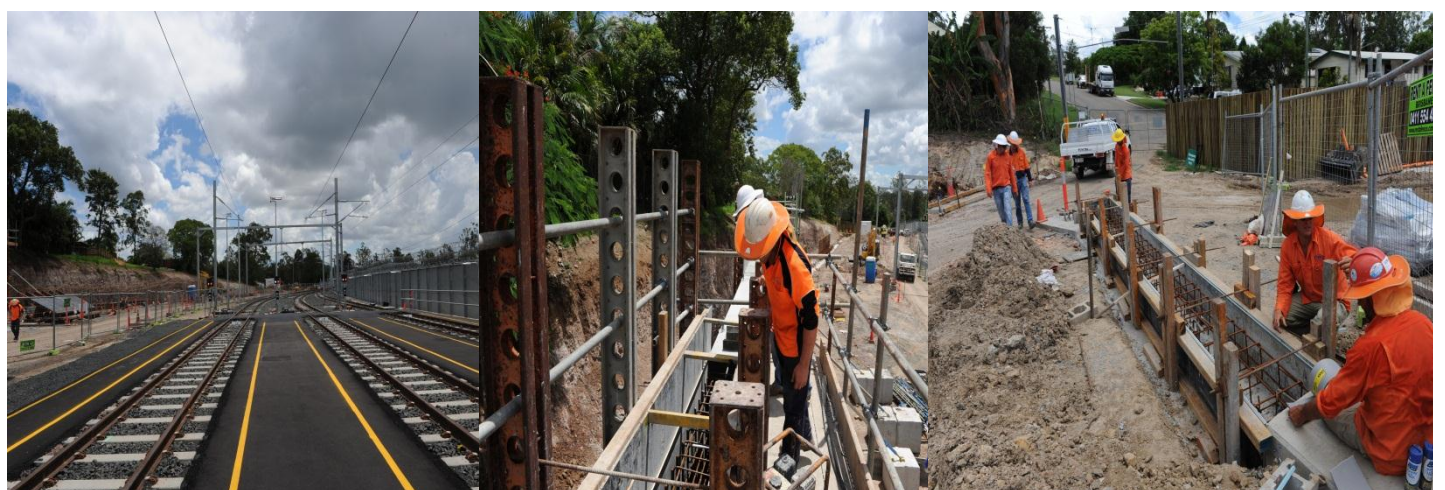
Bottom From Left: Platform raising and track formation preparation; new 9m high retaining wall shaft piled foundation construction
